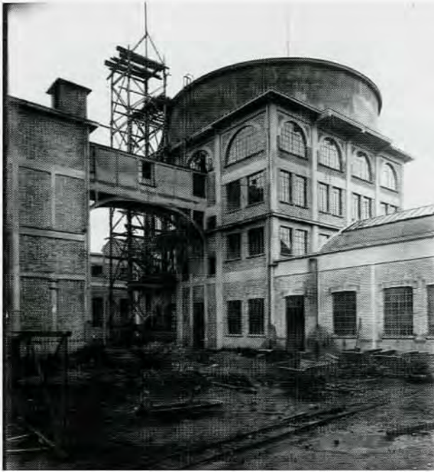
Fig. 3: The water tank building under construction, 1926 (ASR).
