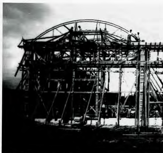
Fig. 6: Arched truss pavilion under construction, 1925 (ASR).
