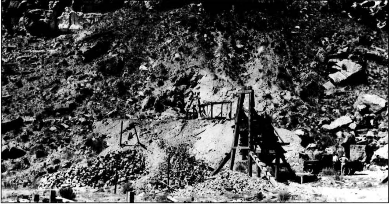
Figure 26. The Hacks Canyon Mine headframe as it appeared in 1948. Photo courtesy of Charles H. Dunning, Arizona Department of Mines and Mineral Resources.
