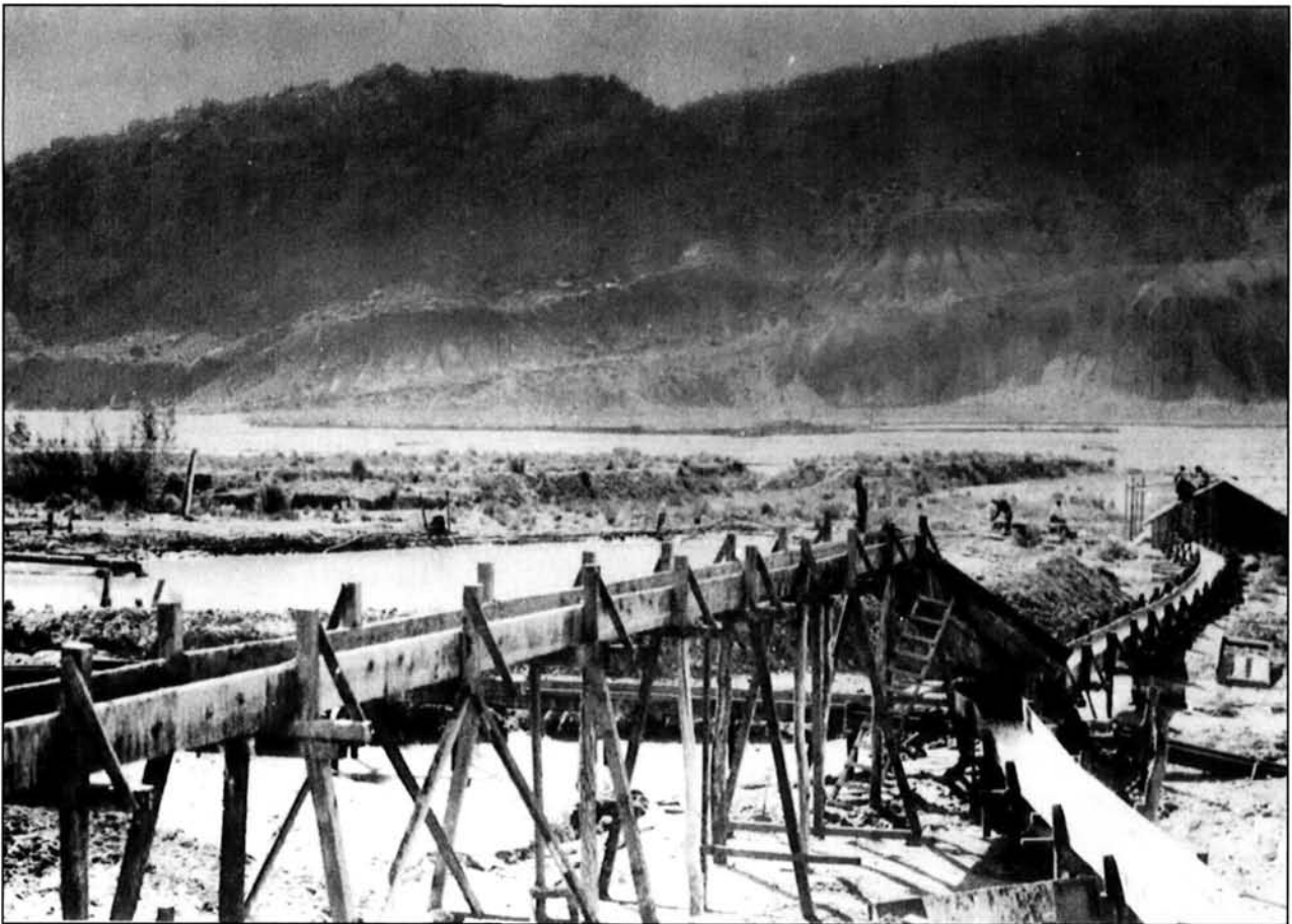
Figure 42. Sluices at the Charles H. Spencer gold placer operation at Lees Ferry, around 1910, leading back toward the Colorado River, and the amalgamator shed. Photo reproduced with permission of the Huntington Library, San Marino, California.
