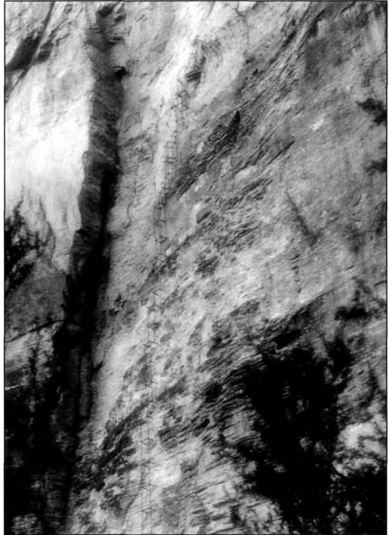
Figure 24. Iron scaffolding is attached to the Redwall Limestone cliff below Mooney Falls on Havasu Creek. The scaffolds once supported wooden ladders that were used to reach a lead, silver, and vanadium mine just out of view at the top of this photo. Most of the wooden ladders were gone by 1970, but several had still been present in the upper half of the scaffolding in 1964. Photo by George Billingsley, 1970.
