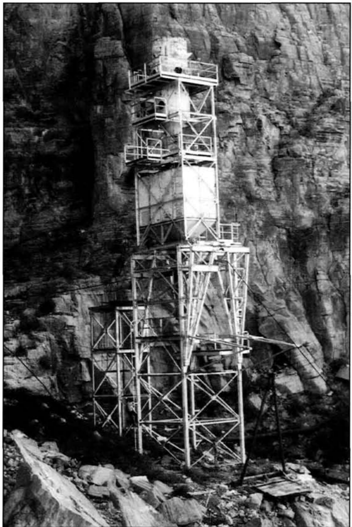
Figure 10. Lower Bat Tower and hopper, just below the Bat Cave. Here guano was loaded into the cable car for transport nearly 10,000 feet across the Canyon to the South Rim (see Figure 11). Photo by George Billingsley, 1976.
