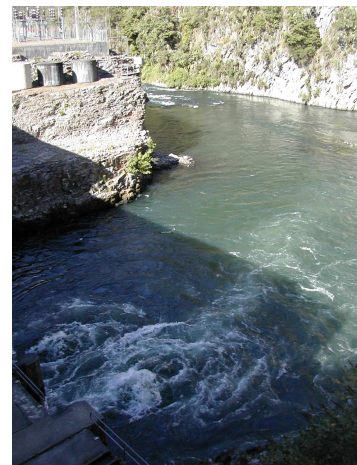
d. Rangitaiki River downstream of Aniwhenua powerhouse
