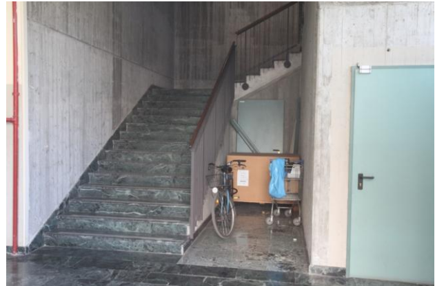
Figure 2. The building's stairway
