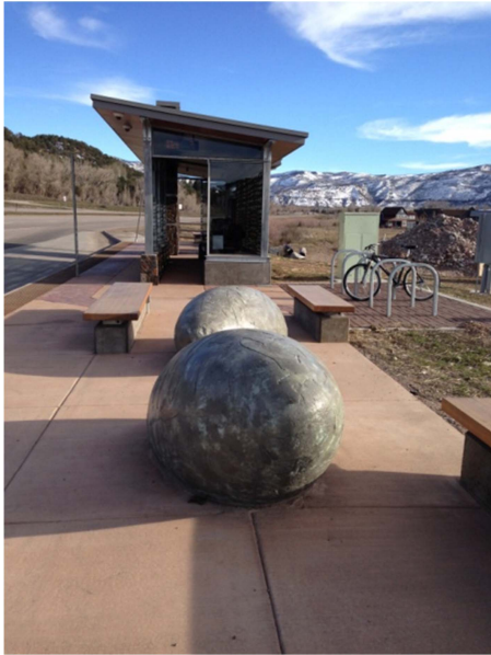
Figure 5 BRT VelociRFTA bus station complete with heaters in the shape of dinosaur eggs.
