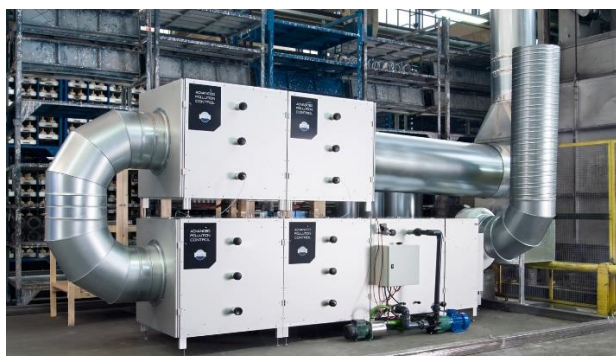
Fig. 2. The Infuser Climatic Gas Phase Advanced Oxidation system being tested at an iron foundry in Germany. The system was effective at destroying benzene, toluene, ethyl benzene and zylene (BTEX).
