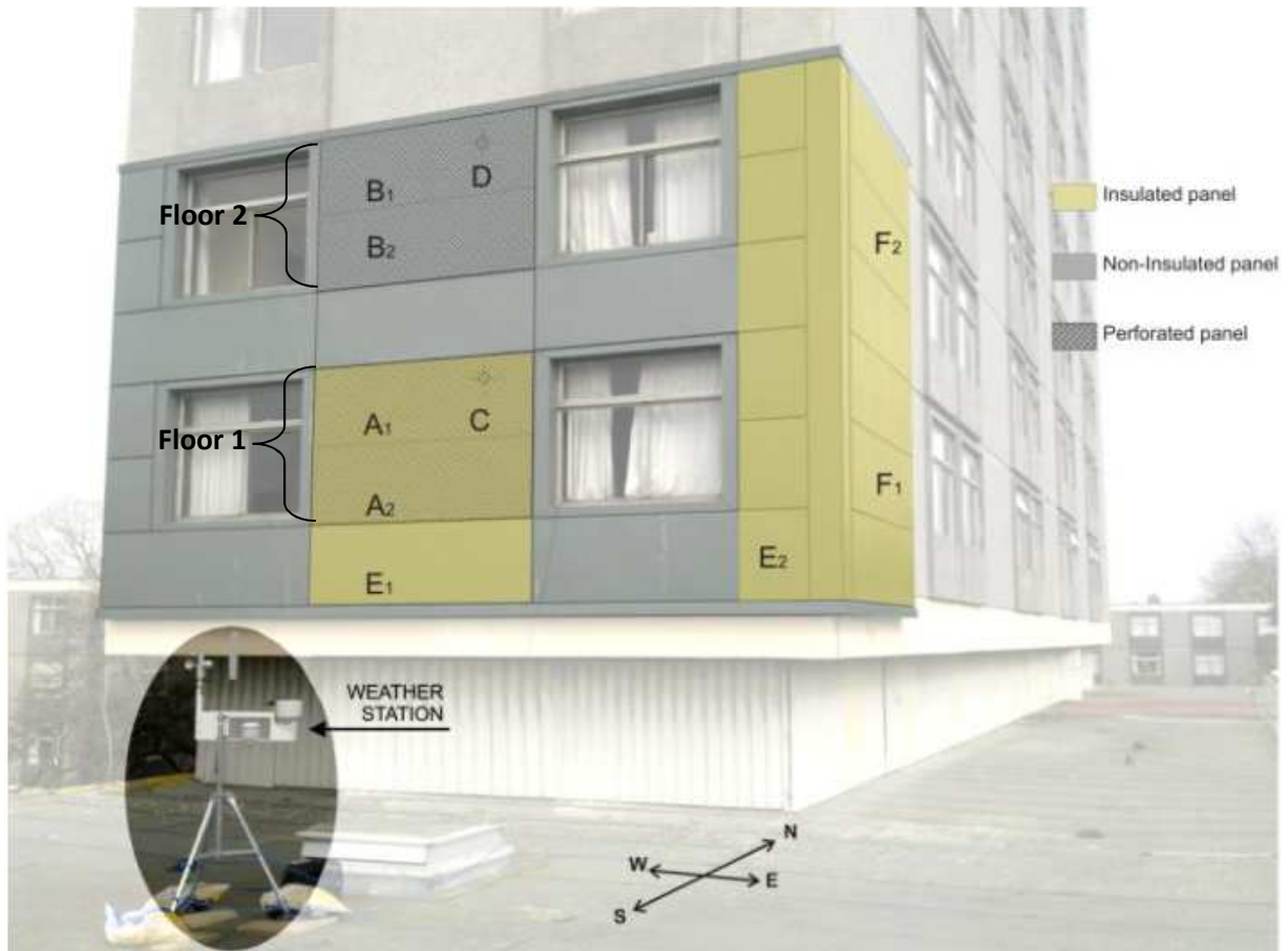
Figure 5 Location of sensors and insulation
