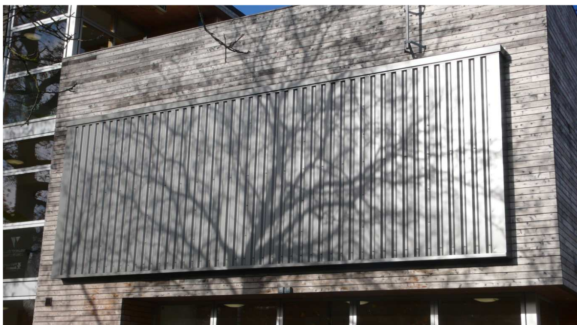
Figure 1 Envelope-mounted profiled TSC installed at the BRE Innovation Park, Watford
