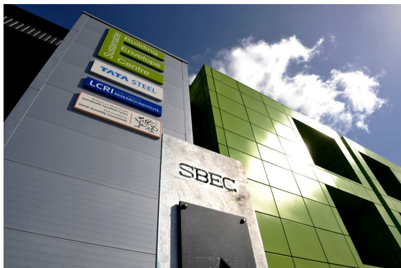
Figure 13 Second generation lime green CP-TSC panels installed on the façade of the Sustainable Building Envelopes Centre in Shotton
