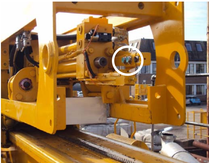
Figure 1. Pile hammer instrumentation for measuring hammer velocity prior to impact (courtesy of Keller Foundations, UK)
