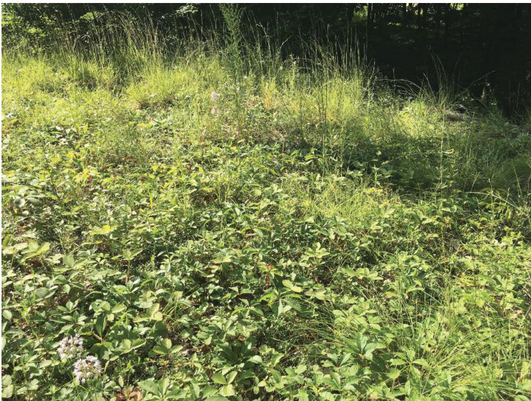
Figure 2. Wellesley College Water Treatment Facility green roof in August 2017.
