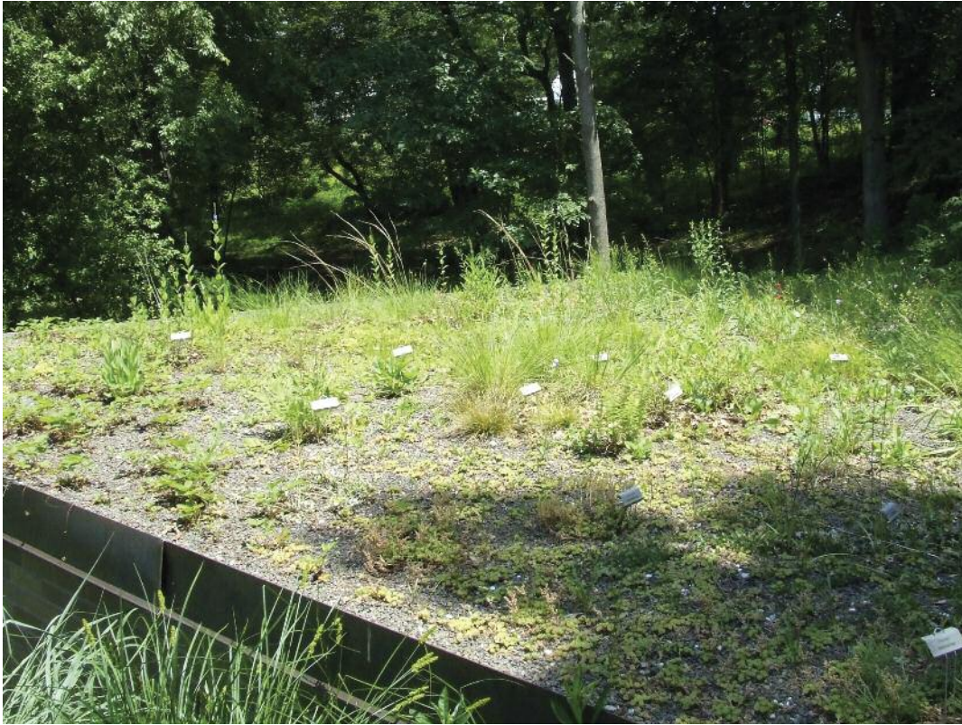
Figure 1. Wellesley College Water Treatment Facility green roof in August 2008.
