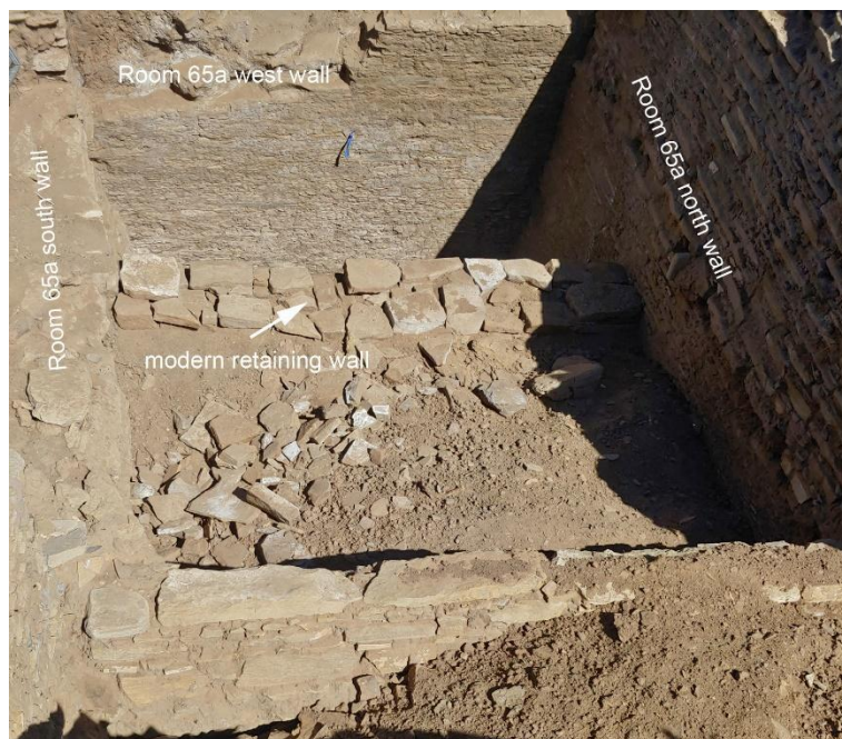
Figure 8. Room 65a with modern retaining wall and spoil.
