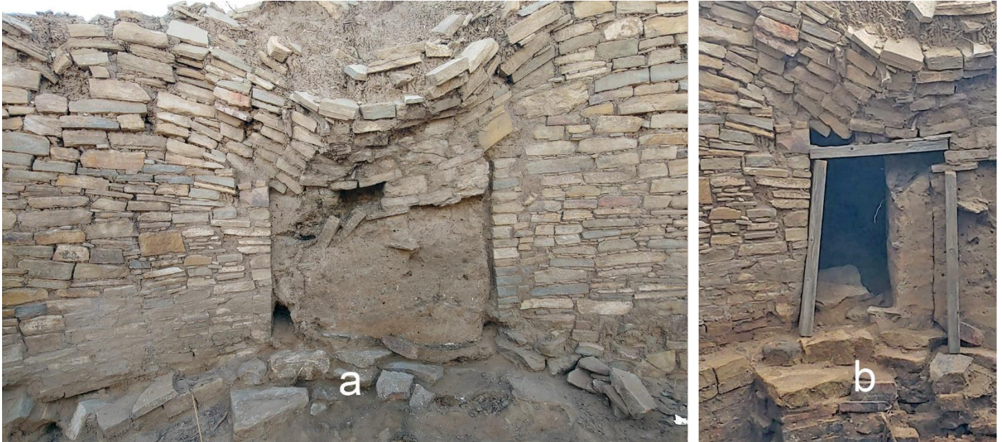
Figure 25. Kiva 32 Feature 1 wall opening. a) collapse; b) test on southeast side.
