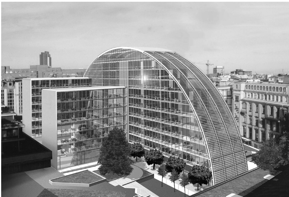
Figure 9: Office building in Hamburg
