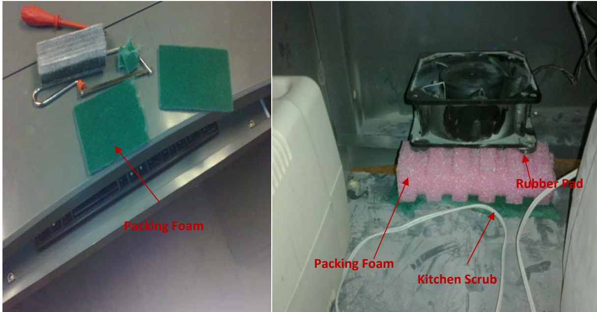
Figure 13 - Three Layered Isolation
