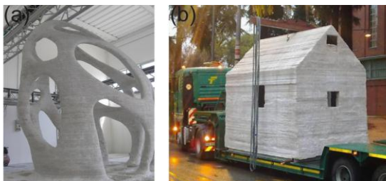
Figure 11. (a): Radiolaria pavilion [20] and (b): the Ferreri house [20] printed by D-shape
