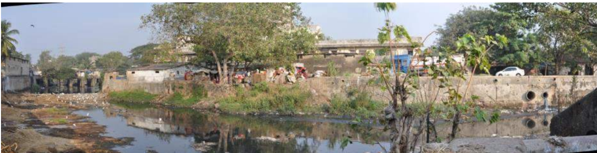
Image 14 Untreated Surface runoff and storm water is released directly into the river.
