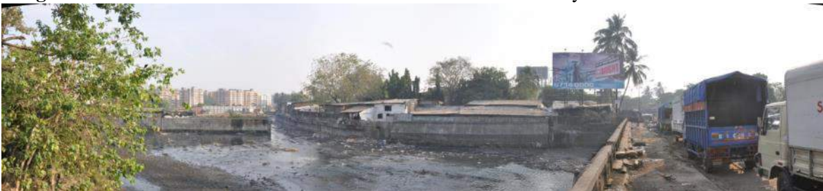
Image 15 Bridges going across the river lack any pedestrian infrastructure and are not properly maintained by the Municipality.
