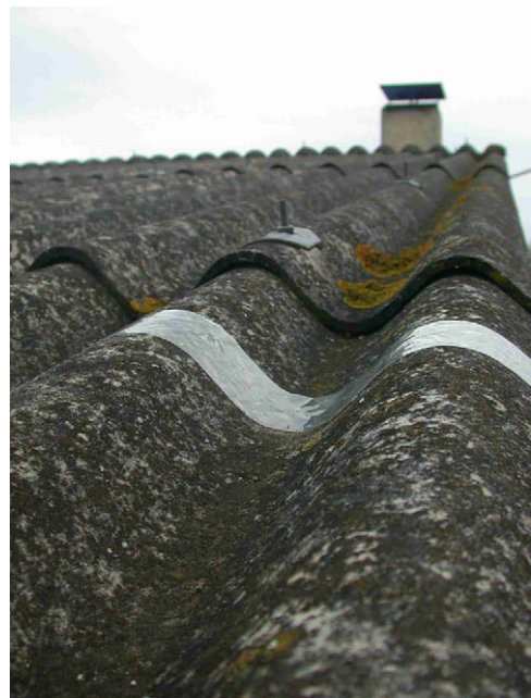
Fig. 4. Example of sampling by pull-up test.
