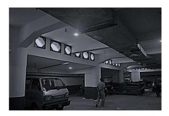
Figure 25. Parking Ventilation based on CO2 level
