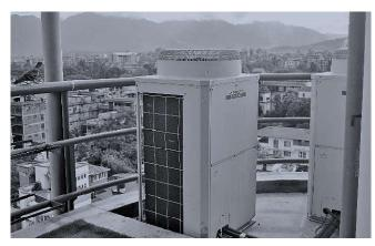
Figure 24. Outdoor Unit of VRV HVAC System
