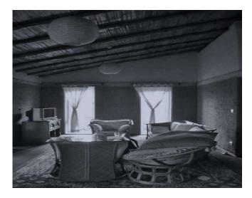
Figure 18. Flattened Bamboo used in roofing
