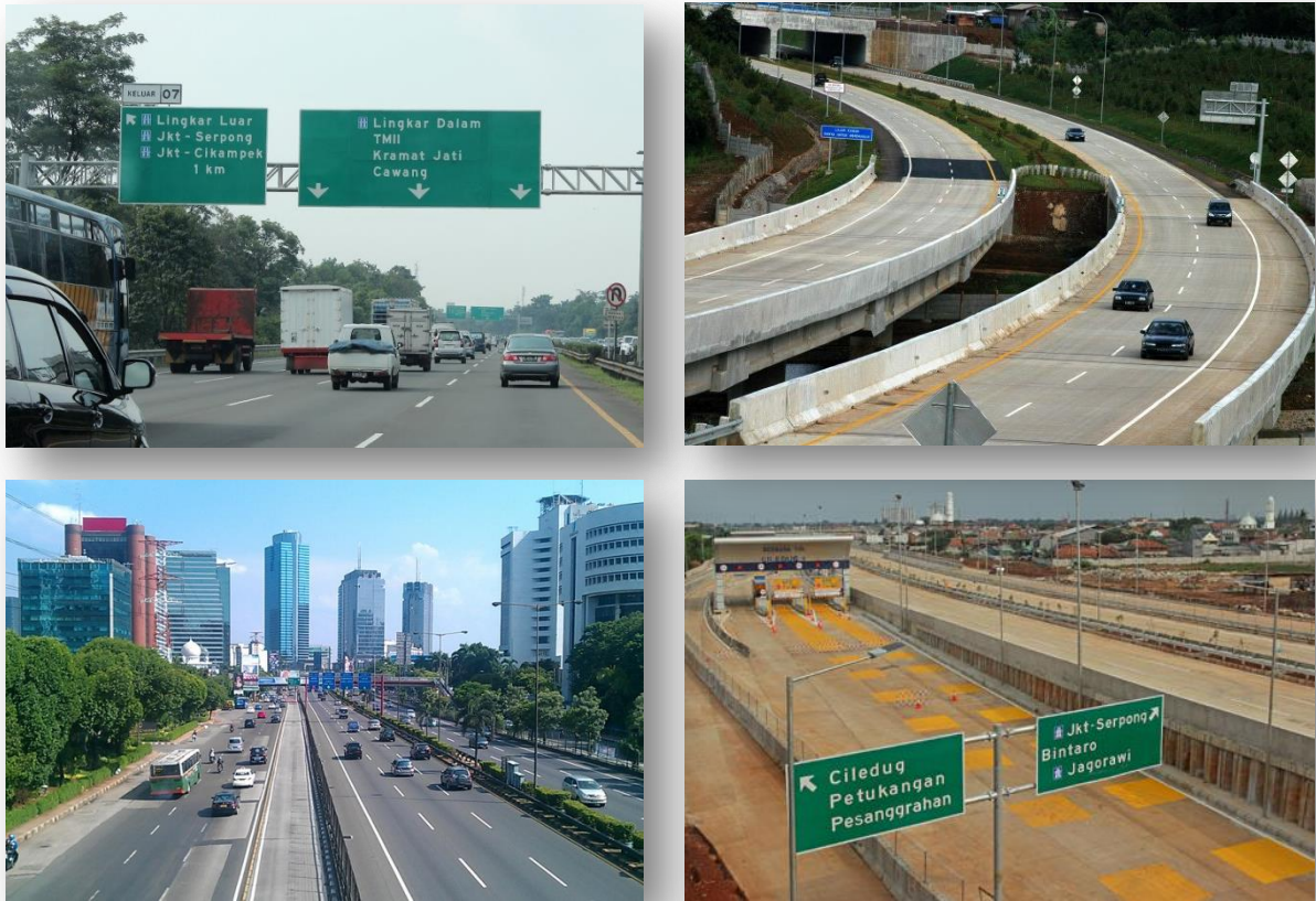
Figure 5 - 17. Transportation infrastructure development in Jabodetabek Megacity: highways and toll roads
