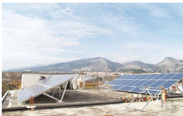
Figure 1: Photo view of the roof of the residence A.
