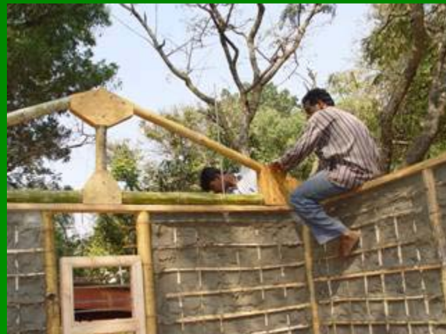
FIXING OF TRUSS
