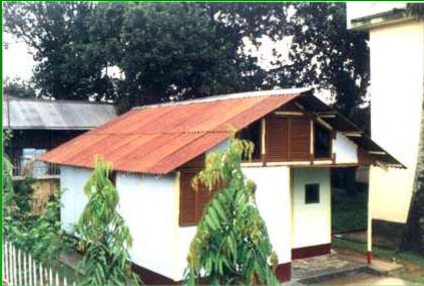
BAMBOO HOUSE BUILT AT AGARTALA
