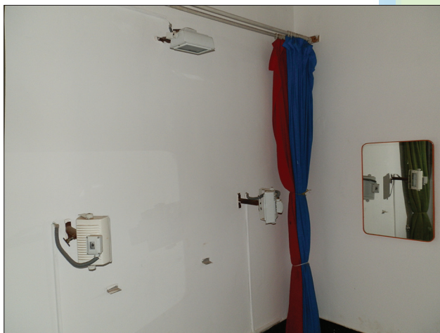
Figure 1: Photography room with wall mounted flood units
