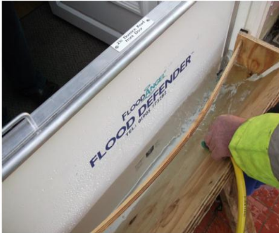
Example of a wet test
