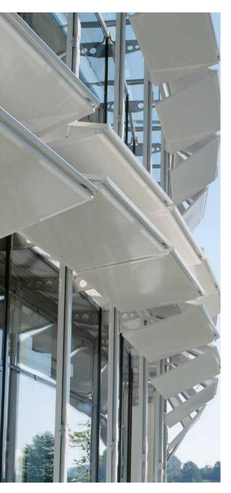
es: a detail of formal as well as technical relevance, because when fully closed, the facade demonstrates its dynamic nature with a subtle ripple.
