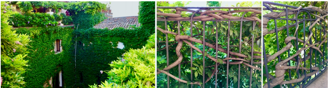
Figure 12. Images of (sustainable, renewable, recyclable) living plant elements applied to architecture; façades which block the direct incidence of the sun with its shadow on the walls, prevent heating in summer, emit oxygen and absorb CO 2 and dust. (Photos: Alberto T. Estévez).
