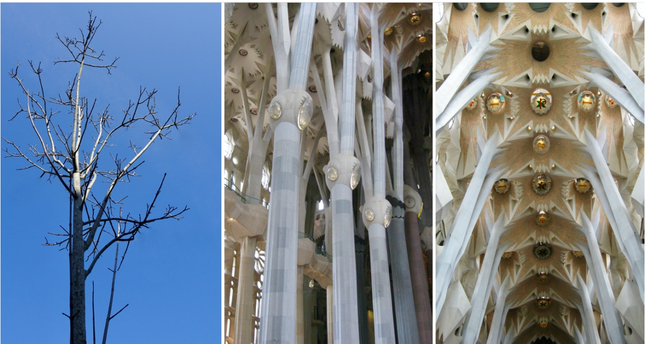
Figure 5. (Below): The pillars spread out like tree branches, following the natural lines of thrust from the structure above. (Photos: Alberto T. Estévez).
