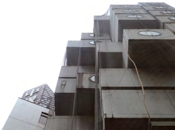
Fig 1 Nakagin Capsule Tower on July 10, 2014 during the author's stay in unit 907B. A makeshift drain pipe hangs from a capsule. The net was placed to protect the pedestrians on the street after the 2011 Tohoku earthquake.
