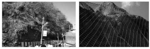
Figure 12: (a) The breast walls provided here cannot function properly during heavy rain induced landslides. These can be replaced with more environment friendly reinforced earth/soils nailed wall, which are not only flexible and cost-saving but also resilient against earthquakes. (b) Application of wire mesh stitched with geonet for protecting one such steep slope. (Photo: Geobrugg)
