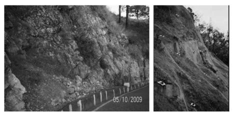
Figure 14: (a) Unprotected rock slope with no proper drainage. (b) Slope protection by nailed wire netting. (Photo: Geobrugg)
