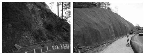
Figure 11: (a) With low height breast wall, slopes along the Yatra track were not protected properly. (b) They can be netted and nailed as per demand of the actual site situation. (Photo: Geobrugg)
