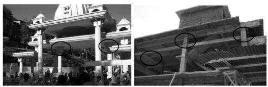
Figure 5: (a) Entrance gate at Katra is likely to be affected in case of earthquake shaking as slender columns and slabs are not supported on load-bearing beam. (b) New constructions have poor quality concrete with thin columns (less than 300 mm wide). Irregular array of secondary beams and columns with floor projections outside, which are extremely vulnerable to earthquake shaking.
