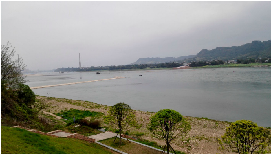
Figure 1. Bank revetment of Nanxi City section of Yibin upper reaches of the Yangtze River.
