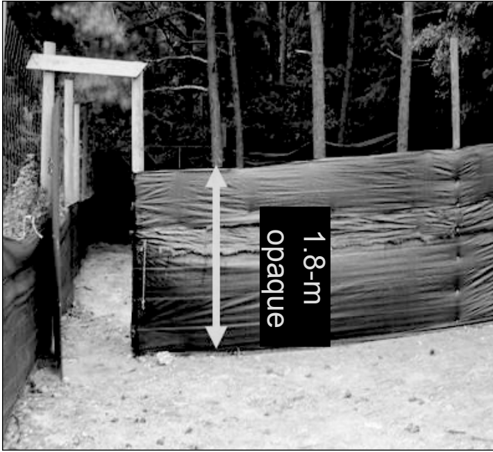
Figure 1. We tested the efficacy of each fence design and height to restrict deer movements in each of 3 treatment areas. This photograph shows an example of a treatment area with test fence and pass-through gate installed.
