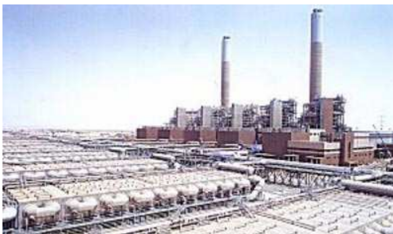
Fig. 20. Multi-stage flash distillation (MSF) desalination plant in Shoaiba currently as the largest in the world [12].
