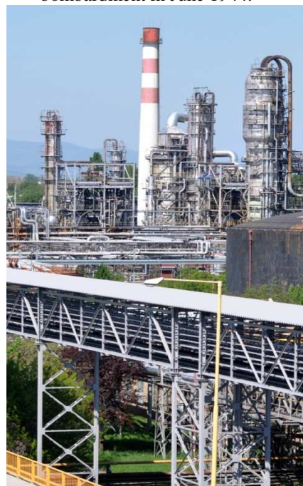
Fig. 18. Atmospheric-vacuum distillation of crude oil in Slovnaft with capacity of 2 mil ton/year.
