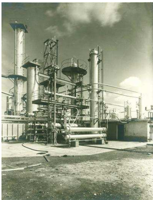
Fig. 15. Atmospheric-vacuum distillation of crude oil in Apollo.
