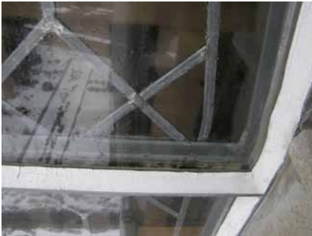
Fig. 2. 'Bonded' protective-glazing system: stained glass fitted in a metal frame together with the protective glazing, installed around 1970. Photo: authors.
