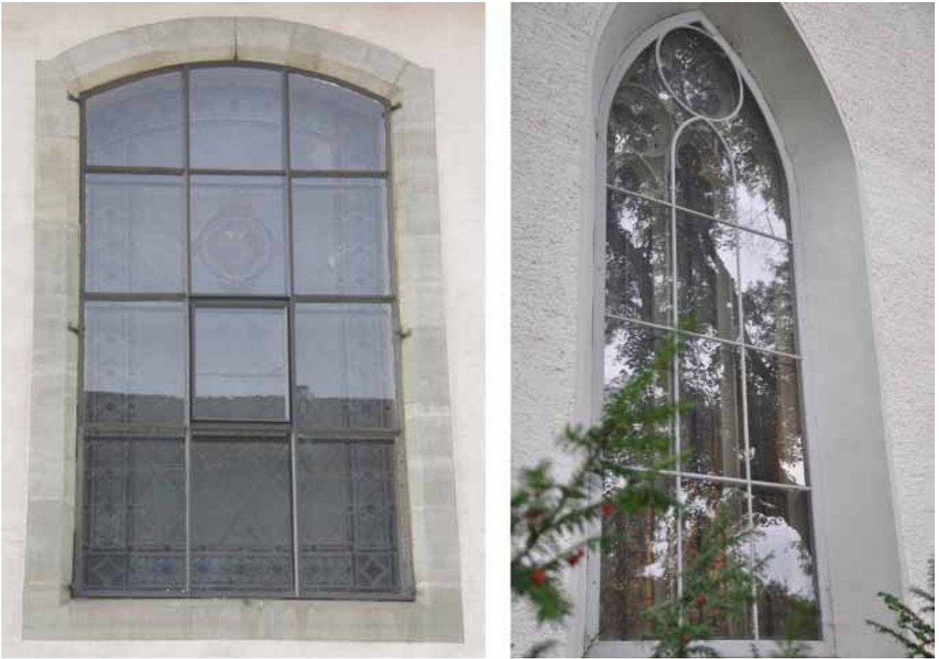
Fig. 1. Unventilated protective glazing fitted in a metal or wood frame: 'Église des Capucins' in Romont, installed around 1950 (left); Parish church of Frauenfeld-Oberkirch, installed probably before or around 1900 (right). Photos: authors.
