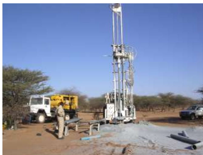
Figure 3: Water Well Drilling in Burkina Faso
