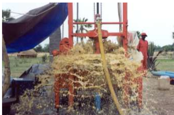
Figure 5: Well Development using Compressed Air
