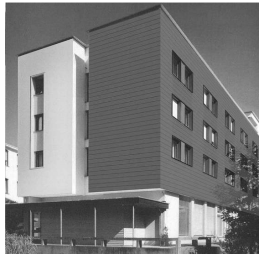
Fig. 4-d. New integration using the SOLABS plank
