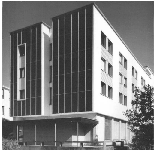
Fig. 4-a. Youth hostel renovation (existing integr.)
