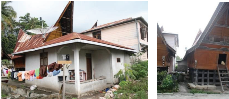
Fig.3. (a) Side Elevation Traditional House (R02 & R03) and its expansion; (b) Front Elevation
