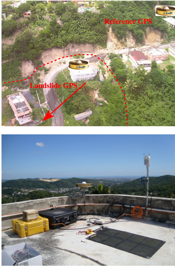
Figure 2. Photos showing the head of the Cerca del Cielo landslide and the continuous GPS monitoring system. The landslide GPS was installed on the roof of a two-story residential building at the head of the landslide. The reference GPS was installed on a one-story resident building outside of the landslide mass. The distance between the landslide GPS and the reference GPS is about 130 meters. Both of the reference and landslide GPS sites are equipped with a Trimble NetRS GPS receiver and a Choke Ring antenna. A weather sensor was also installed at this site in the summer of 2010. Rainfall data from the weather sensor were not used in this study since they only cover a small section of the study period.
