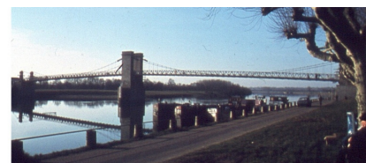
Fig. 1: The Montmerle bridge on the Saône river (France)
