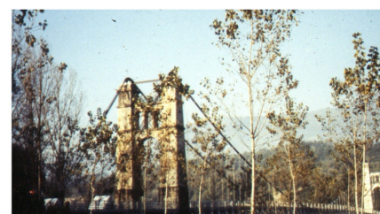
Fig. 2: The Groslée bridge on the Rhône river (France)
