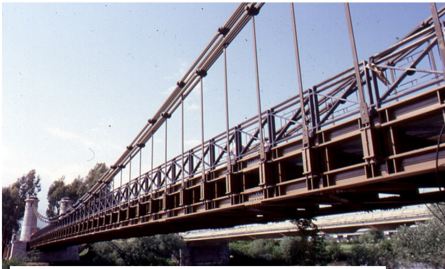
Fig. 5: The new “Real Ferdinando” bridge after erection
