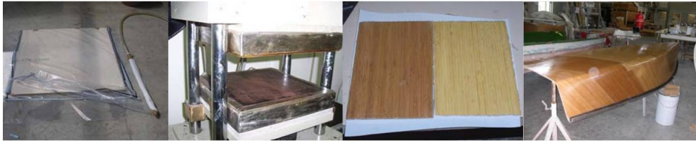
Figure 9. Manufacturing process of bamboo boat hull for water sports activities [40].
