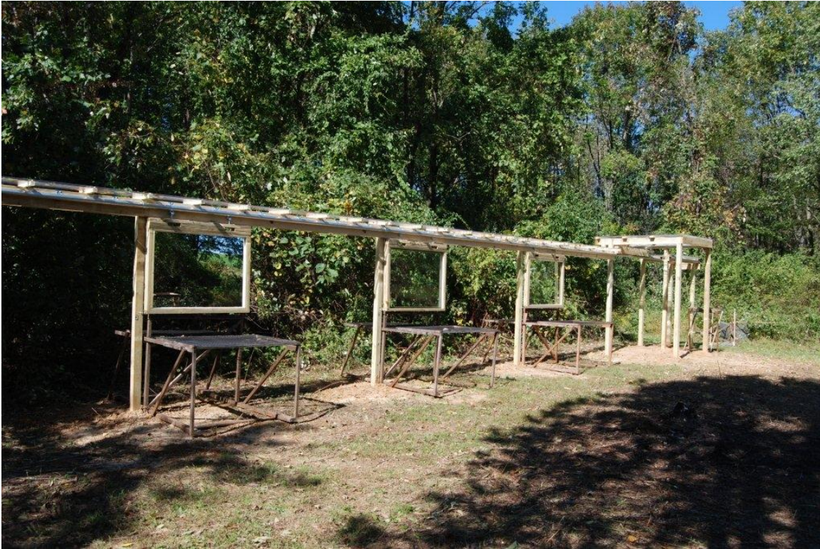
Figure 1. Wooden-framed experimental structure with treatments (window types) in rural Henningsville, Berks County, Pennsylvania, USA.
