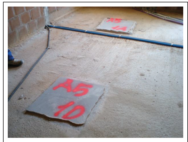
Figure 2. Example of bare floor slab finishing for tapping machine arrangement.
